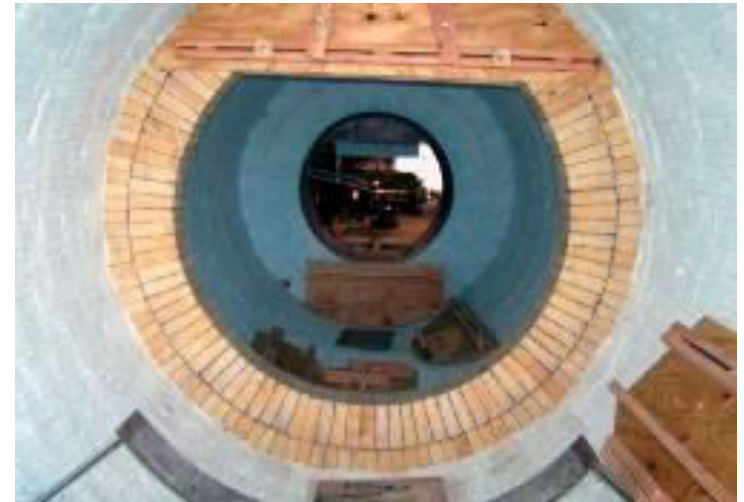
Fig (4 & 5) : Furnace inner lining showing refractory materials
