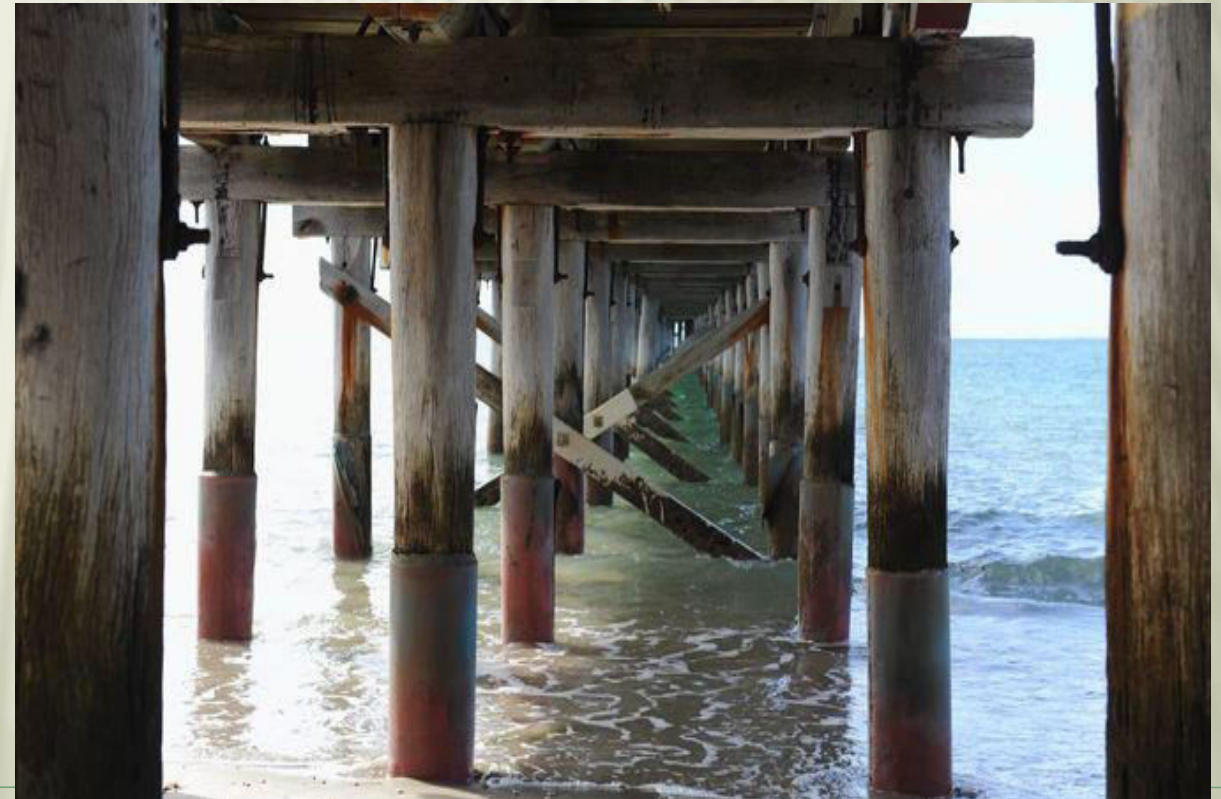
TIMBER-CONCRETE PILE
