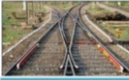
1 in 8 1/2 SINGLE SLIP AT KZI with Malasian Batu Sleepers
