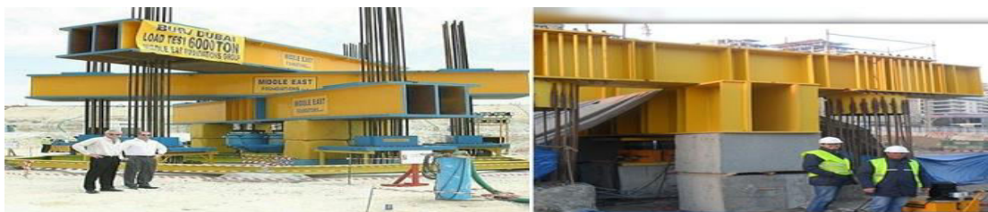
Fig: Vertical load test on piles
