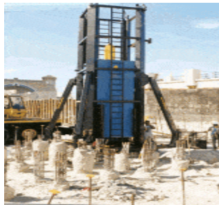
Fig: Pull-out test on piles
