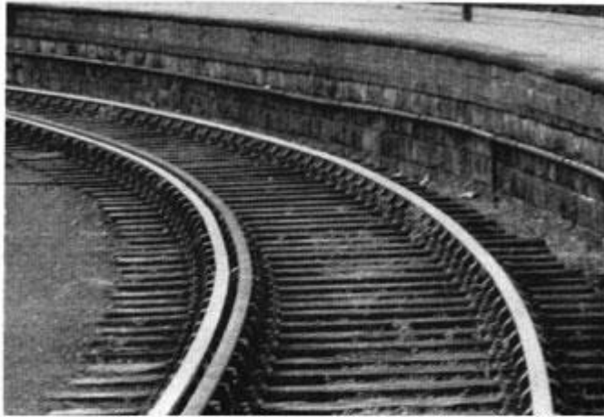
Curves of less than 8 chains radius are fitted with a check rail.
